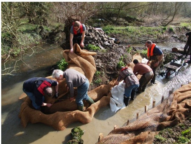
The first Loddon Rivers Week - volunteers and partners building a fish and wildlife bypass channel
